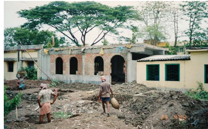
B-10. Construction of general meeting-cum-catering service hall
