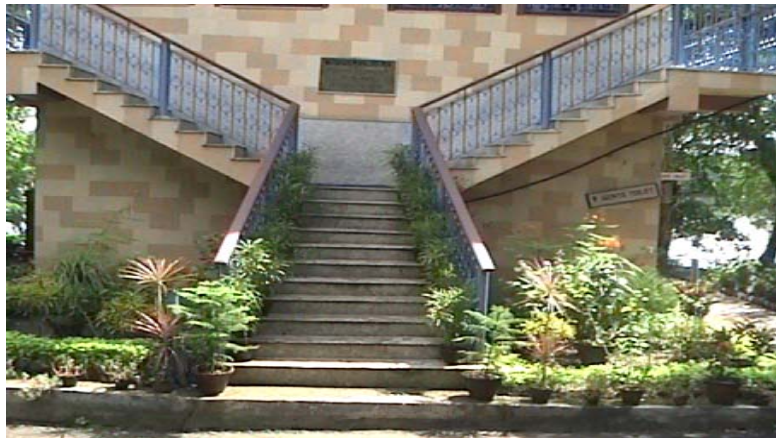
M-35. Bottom view of Society's new office building
