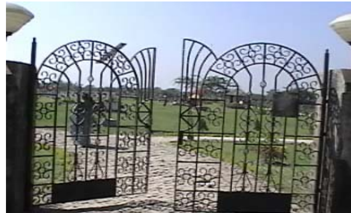
S-30. Entrance to Dhamakhali guest house
