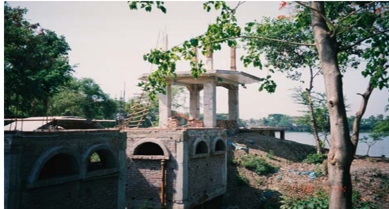
M-21. Folk laboratory being constructed by the Society
