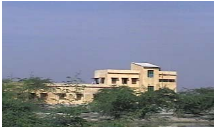
S-25. Marketing complex and training center for SHGs at Damakhali
