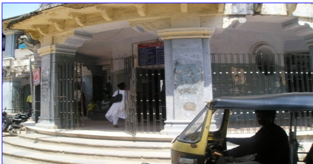
Figure 1: Entrance of Palanpur Civil Hospital
