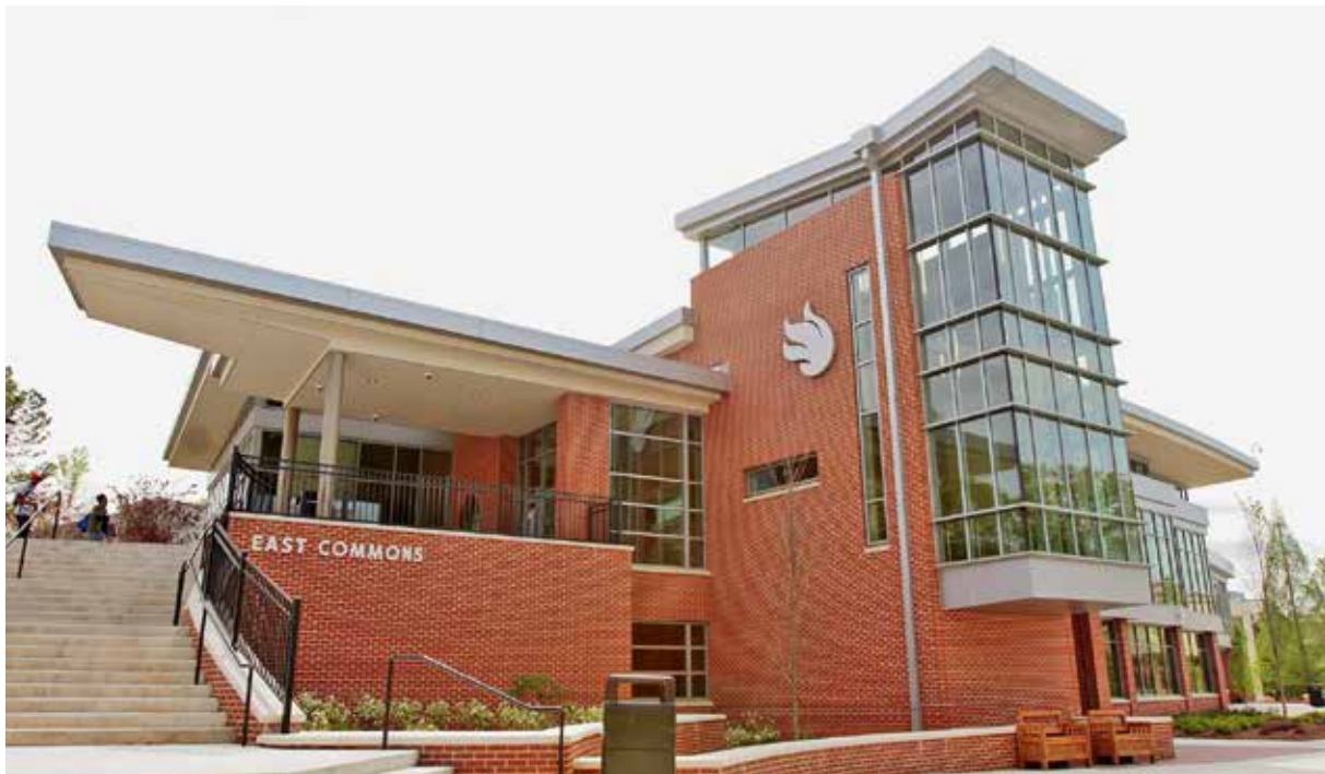
2013a: East Commons: A state of the art campus dining facility. (This was part of my last project, which included a major residence hall shown separately, and the renovation of a small printing facility, also not visible): [~$40 Million.]
